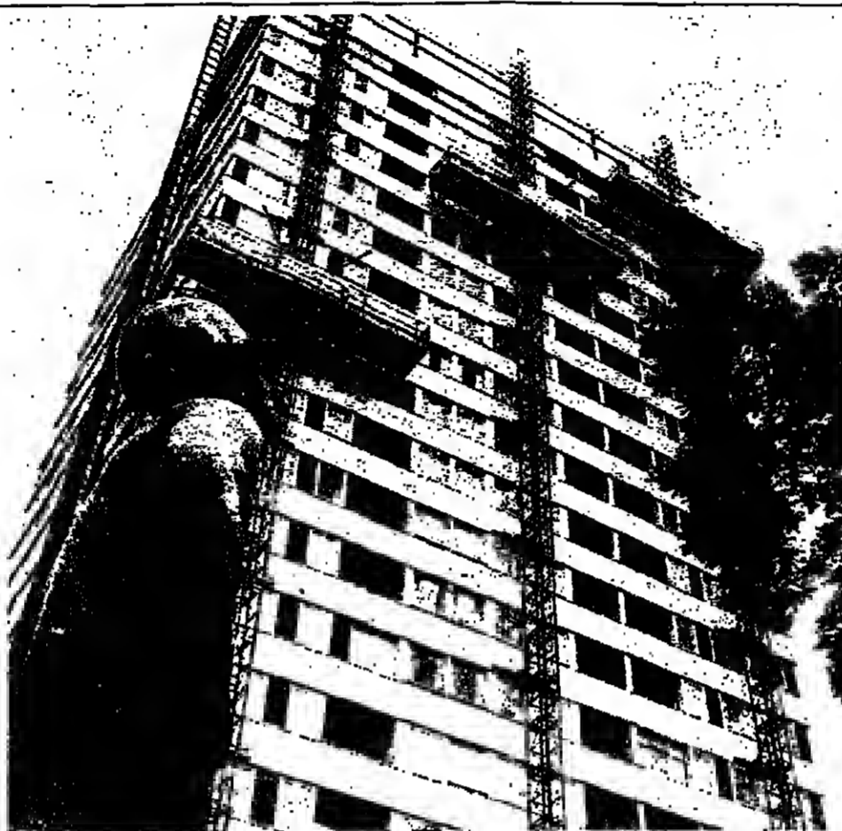
ANSWER TO SCAFFOLDING: Seen here at work on a London building are three "aluminum" a new concept in building industry that is claimed to be cheaper to erect and faster to use than conventional scaffolding. Aluminum is a rack and pinion driven climbing work platform. Steel lattice masts are erected and fixed to the building at 7.5 meter intervals and a platform, with its own electrically-powered drive unit, climbs up the mast. The system allows for rapid changes from one level to another with no inconvenience to the building's occupants.
